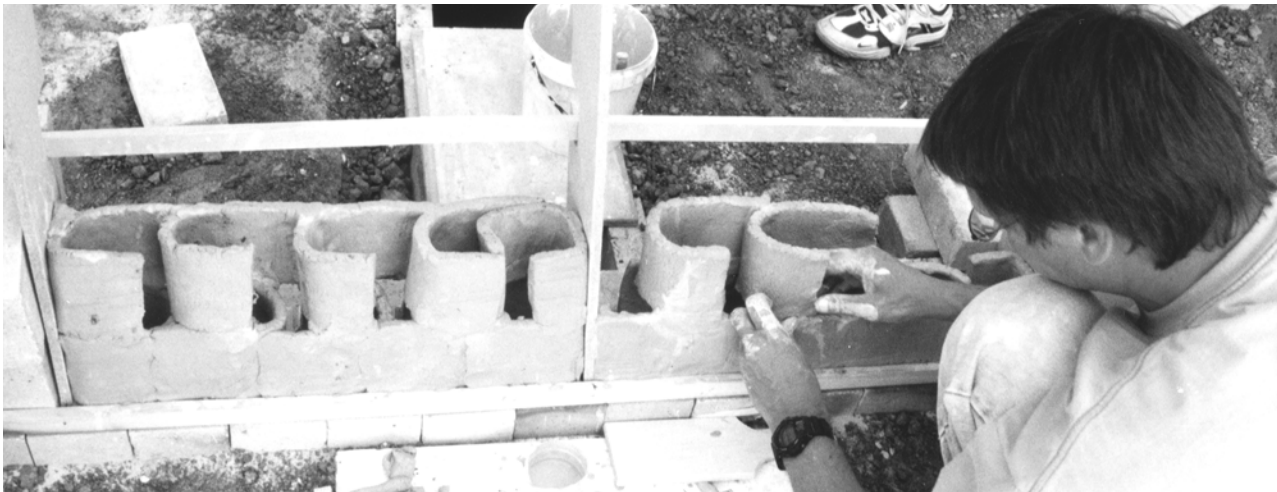
Approximately two tons of clay were needed to build the kiln.
